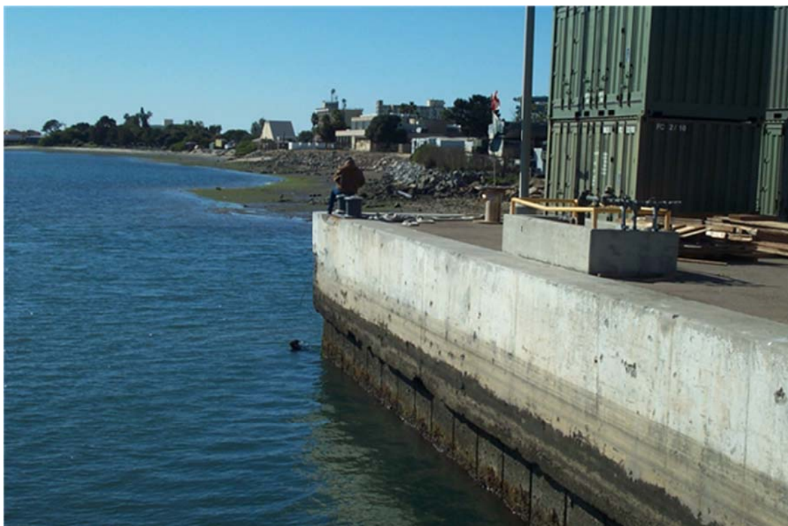
Figure 5-271. Typical Concrete Bulkhead at NAB Coronado.
