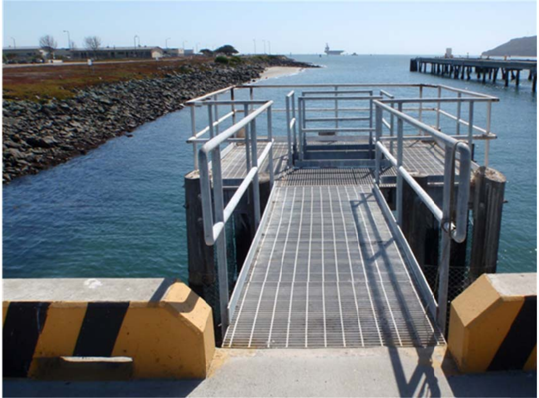
Figure 5-265. Pier Bravo Revetment, NBC.
