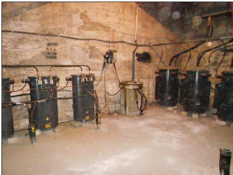
Figure 4-121. The photo shows an electrical vault with older equipment that has exposed connections and is susceptible to flood damage.
