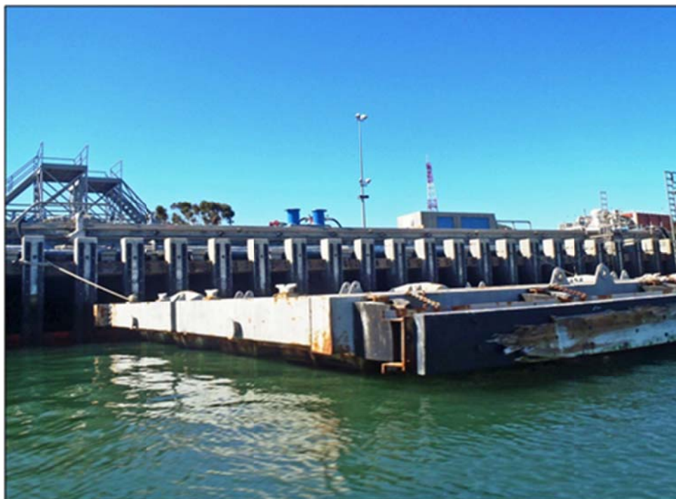
Figure 5-254. An aircraft carrier separator is a floating platform that provides clearance between the aircraft carrier and the wharf fender system, shown moored at Carrier Wharf Berth Kilo, NBC.
