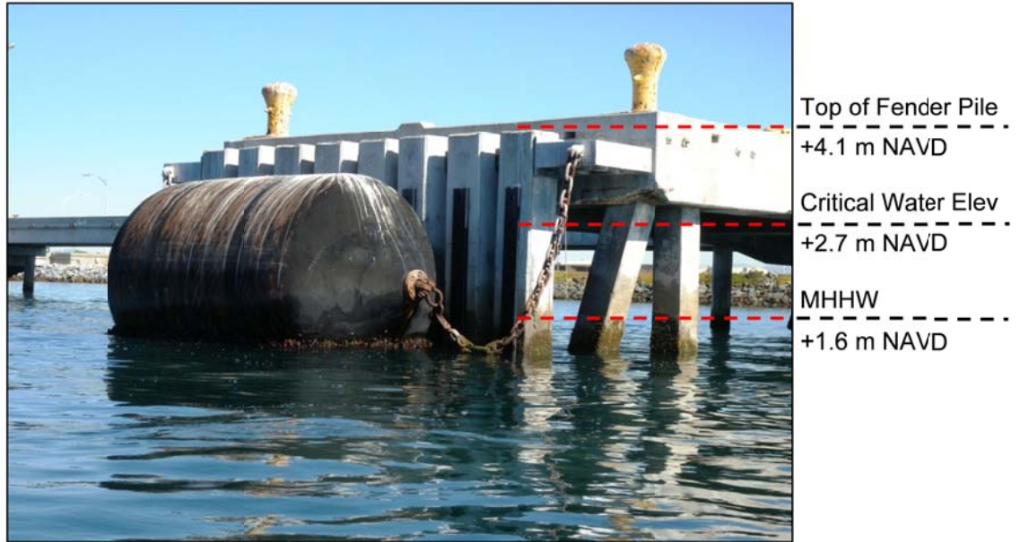
Figure 5-245. View of floating fender and concrete piles at Ammunition Pier Bravo, NBC. This system is vulnerable to “roll-over” with 0.5 m of SLR.
