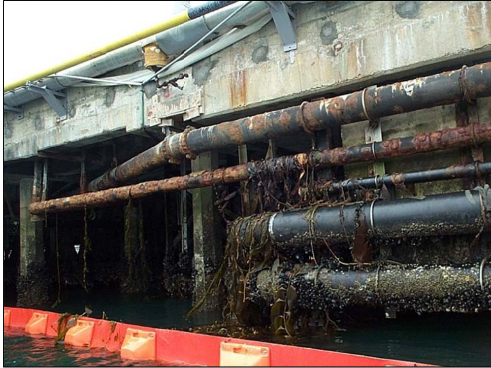
Figure 4-109. Pier with utility pipes located below deck in the tidal zone. The pipes are submerged during high tides and collect kelp and other debris.
