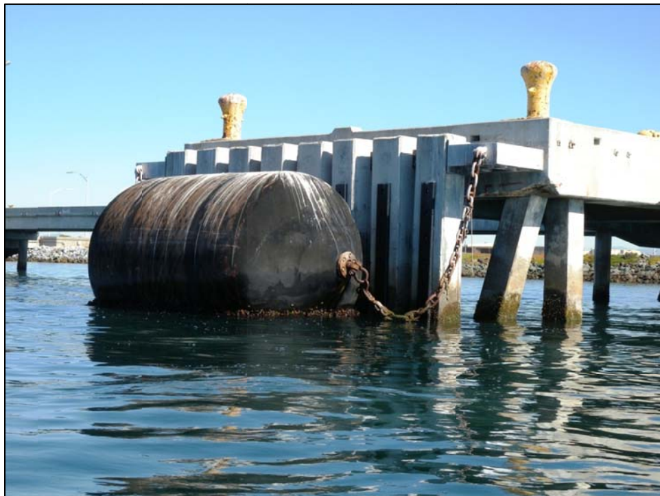
Figure 4-104. Typical pier fender system with floating fenders and concrete reaction piles at a close spacing for bearing.
