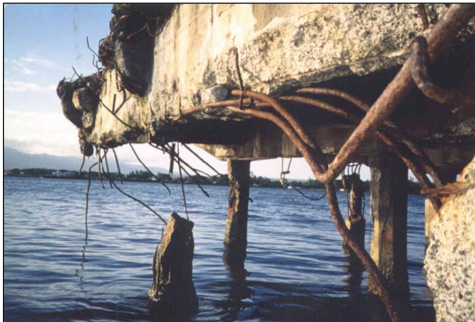
Figure 4-113. Waterfront structure that has excessive deterioration from chloride contamination and corrosion of the reinforcing steel (Courtesy Blaylock Willis and Associates).
