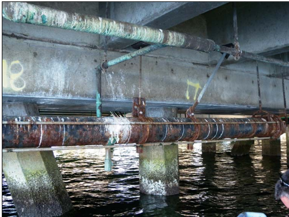
Figure 4-110. Pier with water pipe located below deck. The pipe and hangers may not be designed for wave and current loading.
