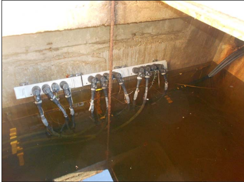
Figure 4-120. The photo shows a below-grade electrical vault partly full of water. A connection panel is visible above the water. The vault remains operational.
