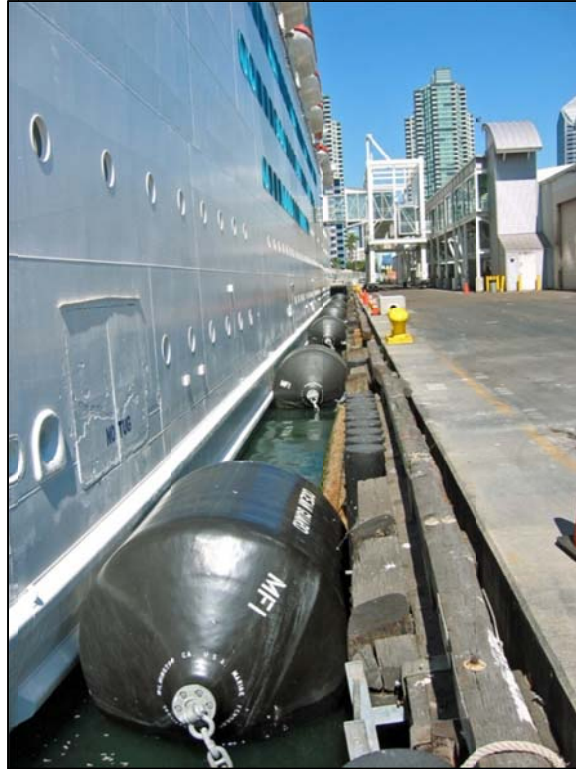
Figure 4-105. Foam filled fenders shown at high tide. With less than 1.0-m of SLR, "roll-over" could occur.
