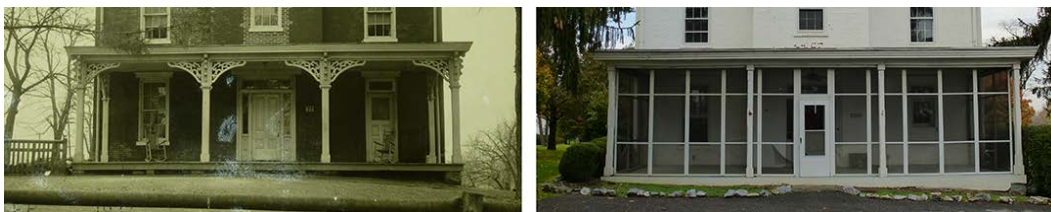
Figure 59. A comparison of the front porch from the 1920s (NARA) to present-day (ERDC-CERL, 2012).
