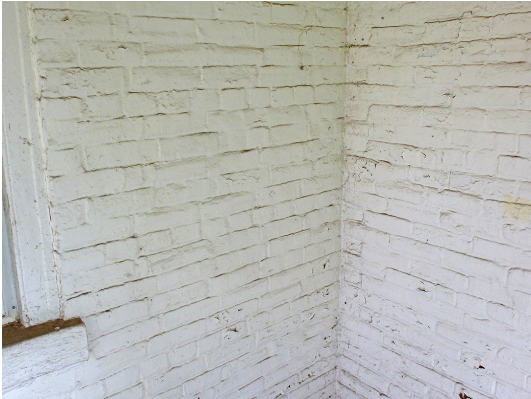
Figure 53. Detail of the brickwork and mortar joints (ERDC-CERL, 2012).
