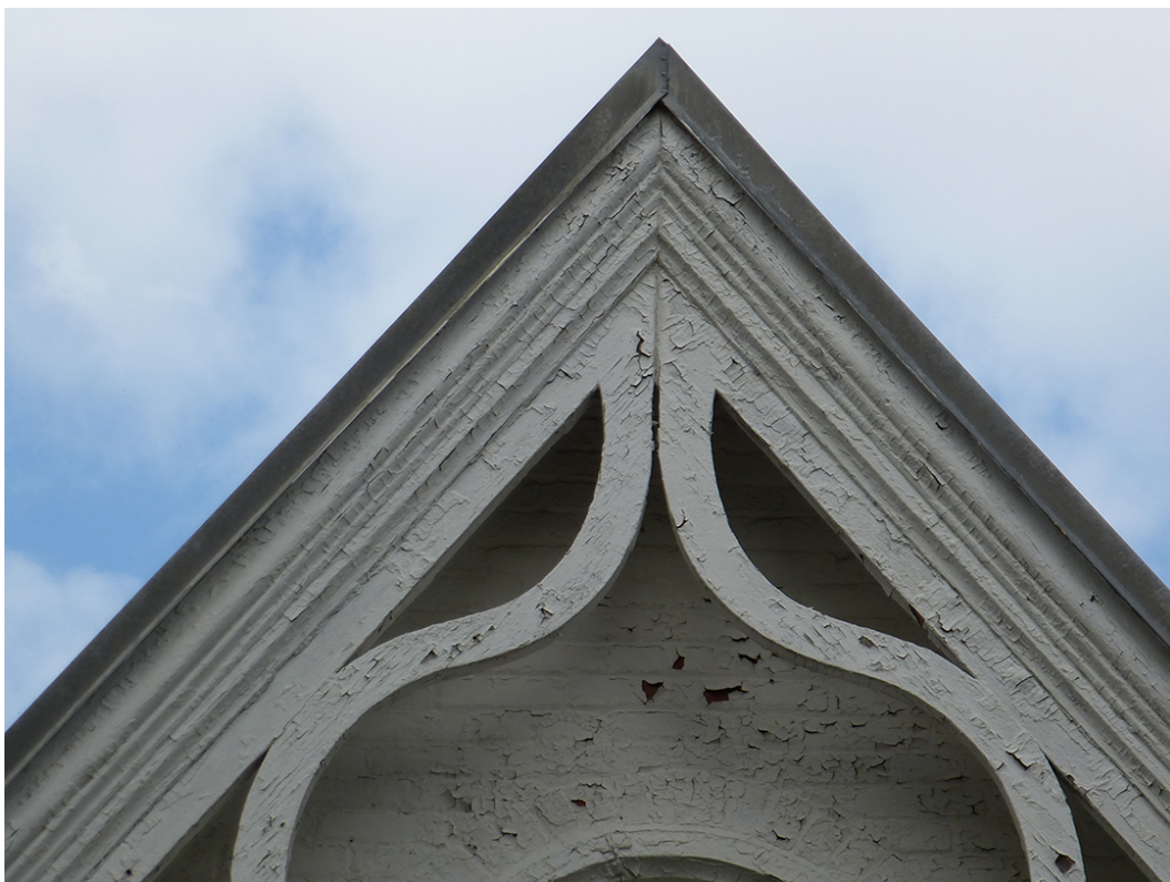
Figure 54. Detail of the rake boards on the front gable (ERDC-CERL, 2012).
