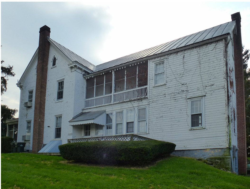
Figure 19. East façade in 2012 (ERDC-CERL, 2012).
