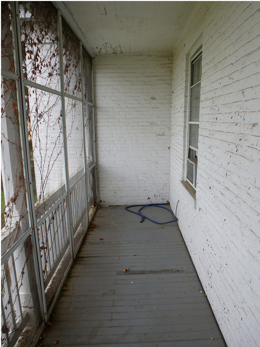
Figure 45. Second floor of the east porch on the ell (ERDC-CERL, 2012).
