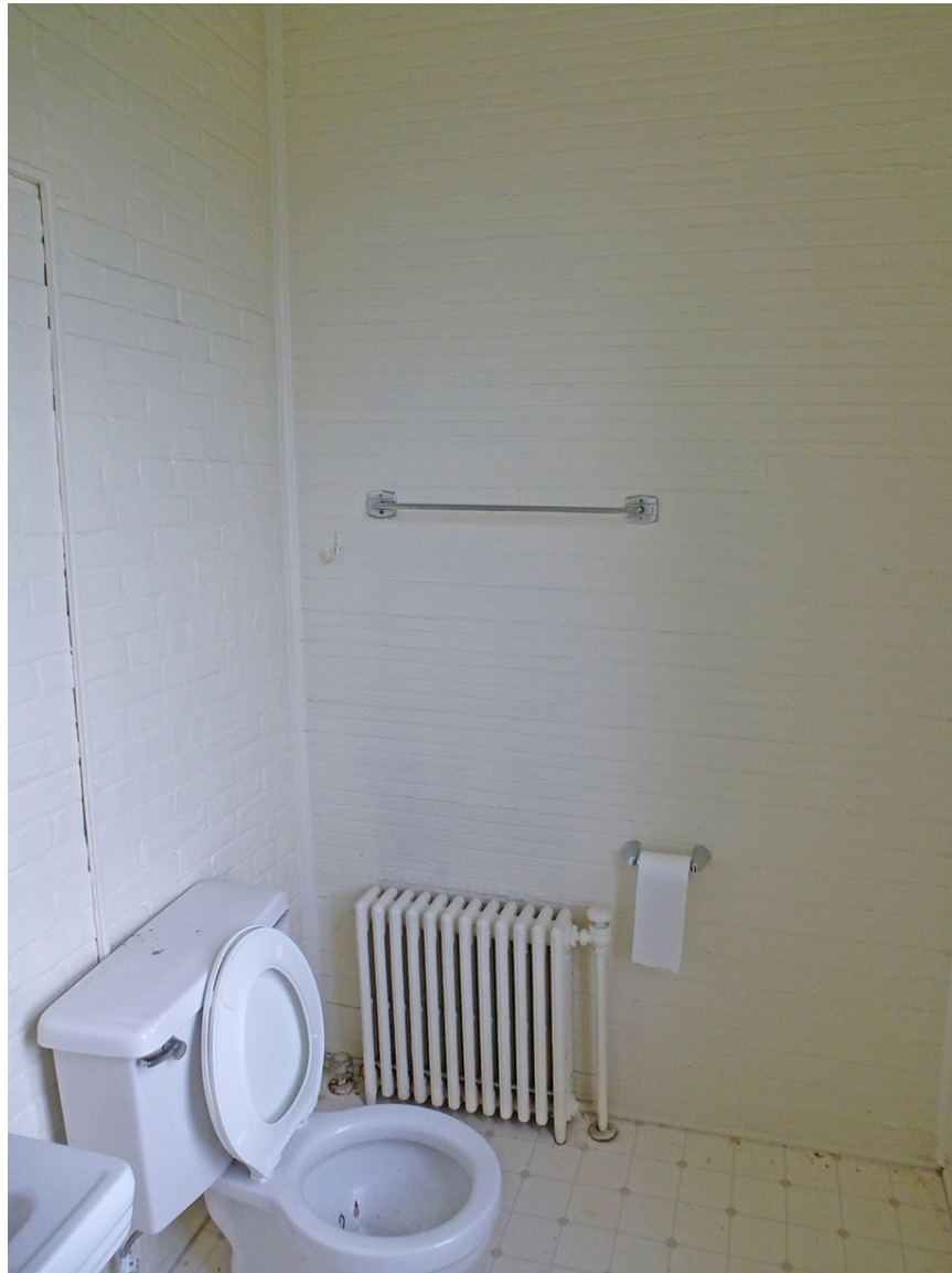
Figure 39. Bathroom on the north porch (ERDC-CERL, 2012).
