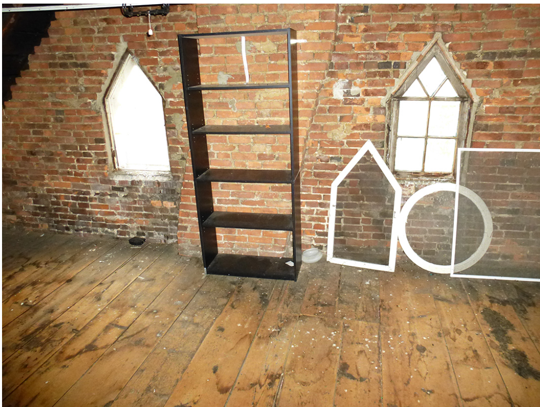
Figure 32. Storage room, attic level of south side of duplex (ERDC-CERL, 2012).
