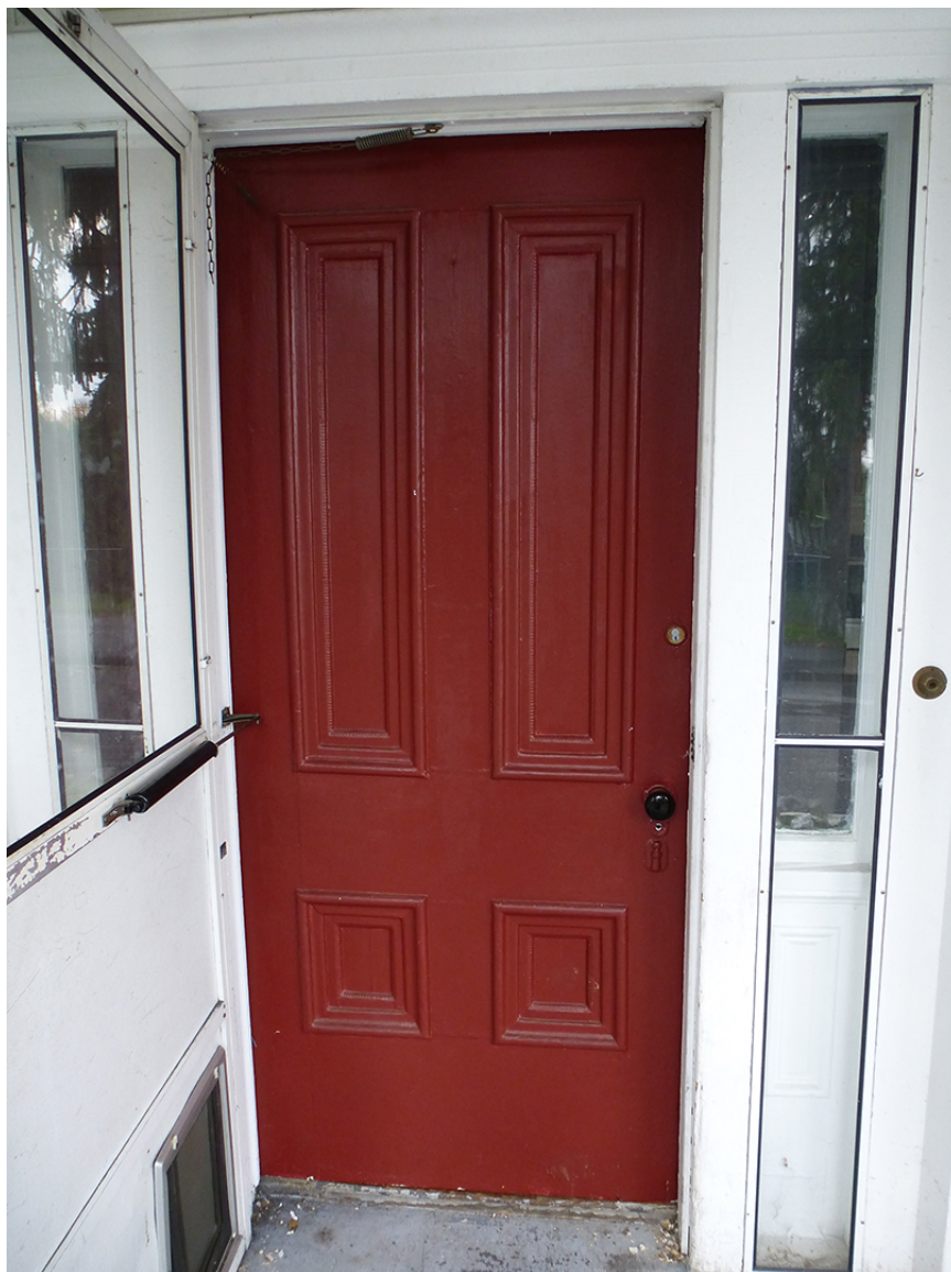
Figure 20. Front door in 2012 with sidelights (ERDC-CERL, 2012).
