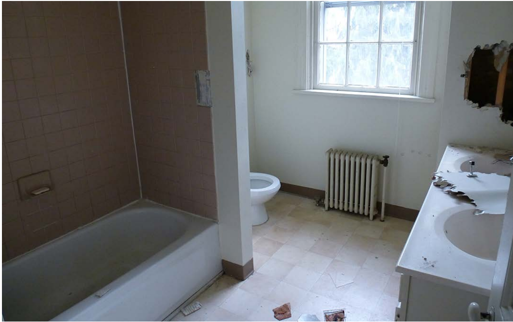
Figure 29. Second-floor bathroom, south part of duplex (ERDC-CERL, 2012).
