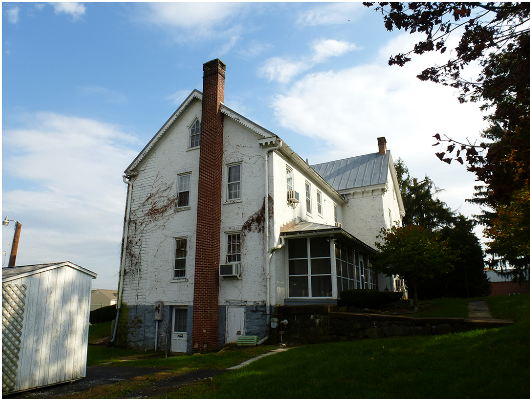
Figure 18. North façade (rear) in 2012 (ERDC-CERL, 2012).
