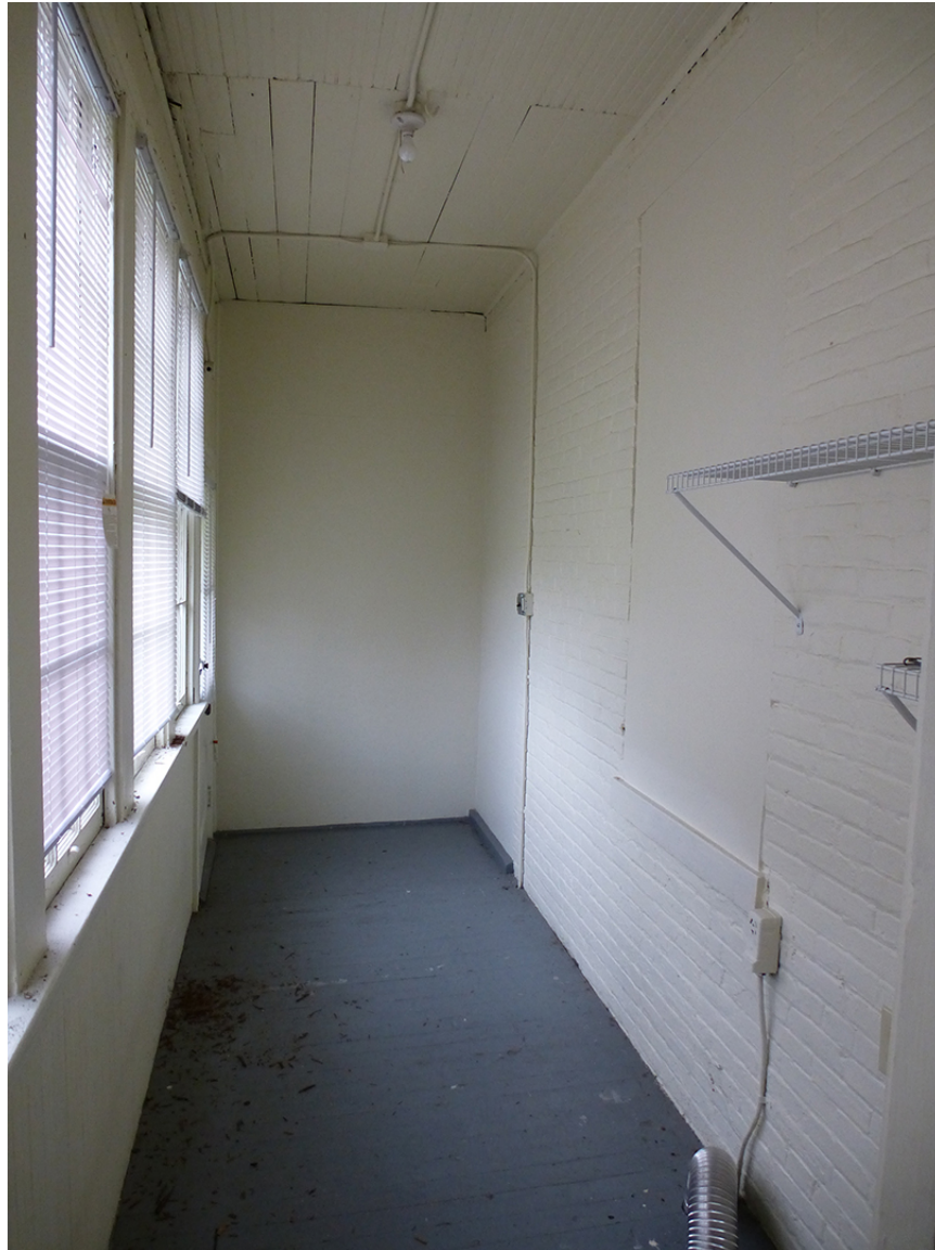
Figure 38. North porch of the ell (ERDC-CERL, 2012).
