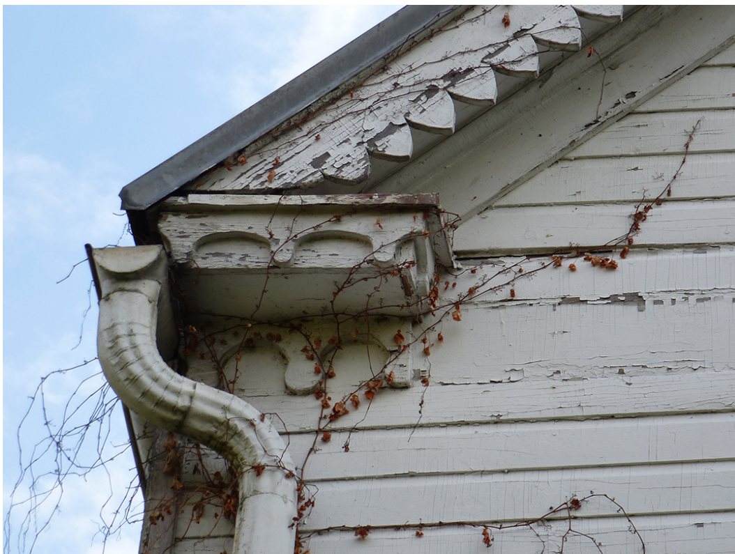
Figure 56. Detail of the rake boards on the ell gable (ERDC-CERL, 2012).
