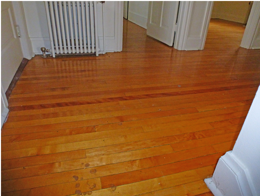
Figure 40. Second-floor hallway of the ell (ERDC-CERL, 2012).
