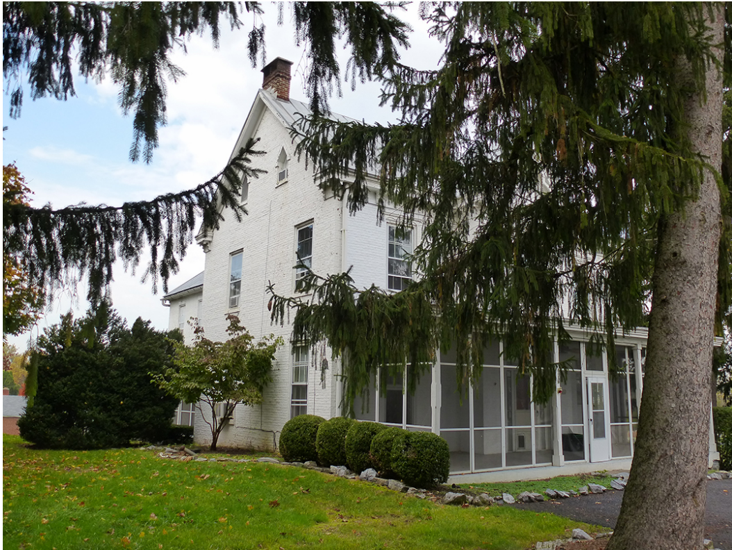
Figure 17. An oblique of the west and south façades in 2012 (ERDC-CERL).
