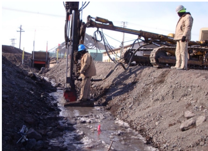
Figure A2. Using a drill rig to install the sensors.
