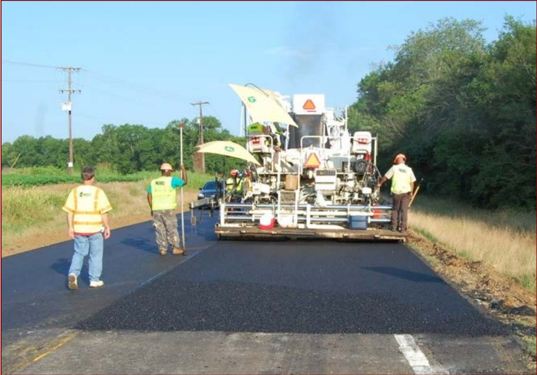
Figure 4. Test Site 2 at Okolona, Mississippi.
