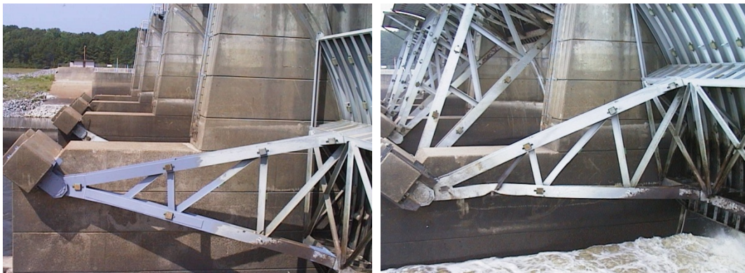
Figure 11. Tainter gate with strut arm damage due to a barge impact and after the repairs were made.
