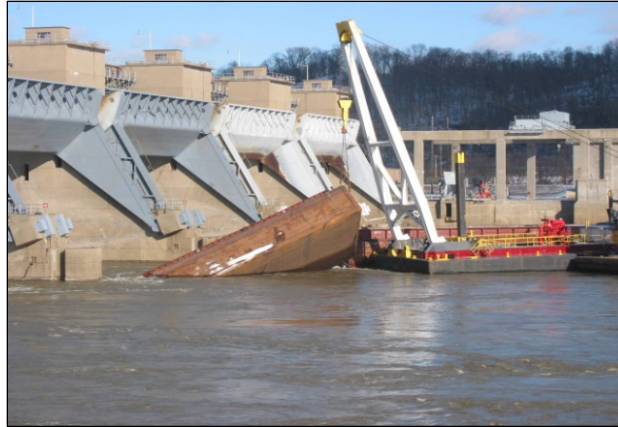
Figure 10. A Belleville Locks & Dam Barge Impact.
