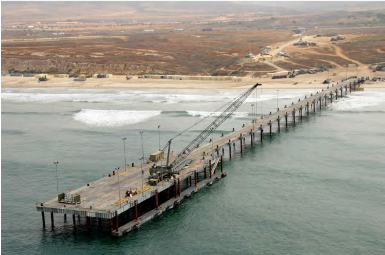
Figure 4 - Elevated Causeway (ELCAS) Photo 25
