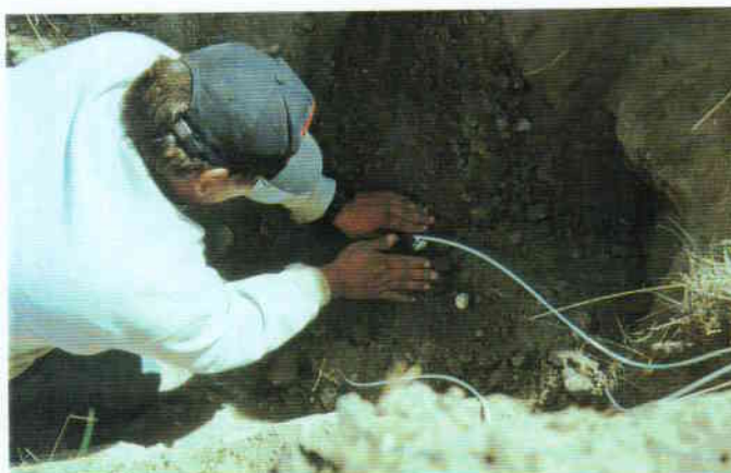
Figure 16. A shaped-charge challenge on a projectile is being tamped in place using soil to minimize scattering of shrapnel during detonation.
