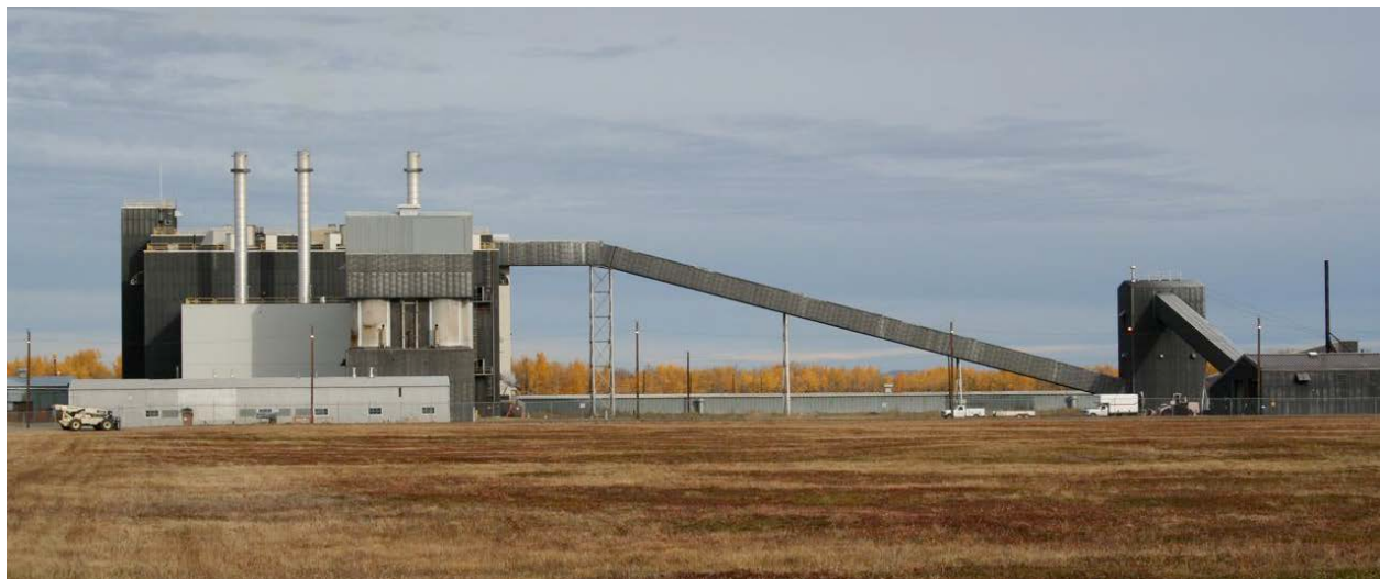
Figure 2. Clear AFS Power Plant, Facing North.
