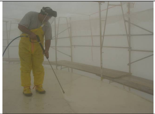
FIGURE 12. Surface Preparation by Water Blasting.
