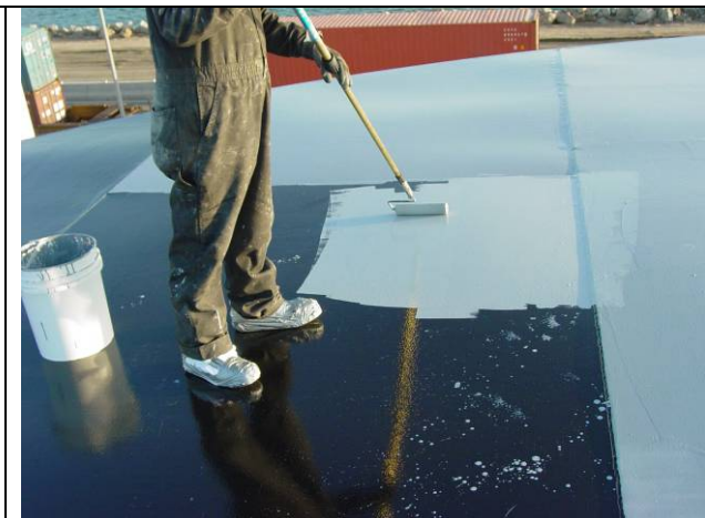
FIGURE 14. AZT Topcoat Applied by Rollers on Tank 2001 roof.
