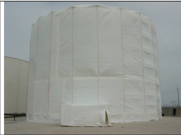
FIGURE 11. Containment Plastic over Scaffolding on Tank 2003.
