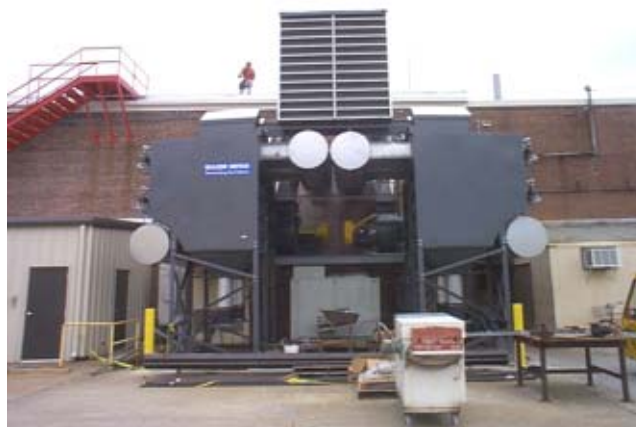
Figure 3. Air Handler and Dust Filter Installation at NADEP-CP.
