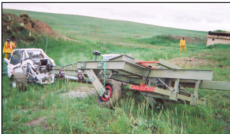
Figure 13. STOLS Inside the Demolition Pit at Lowry.
