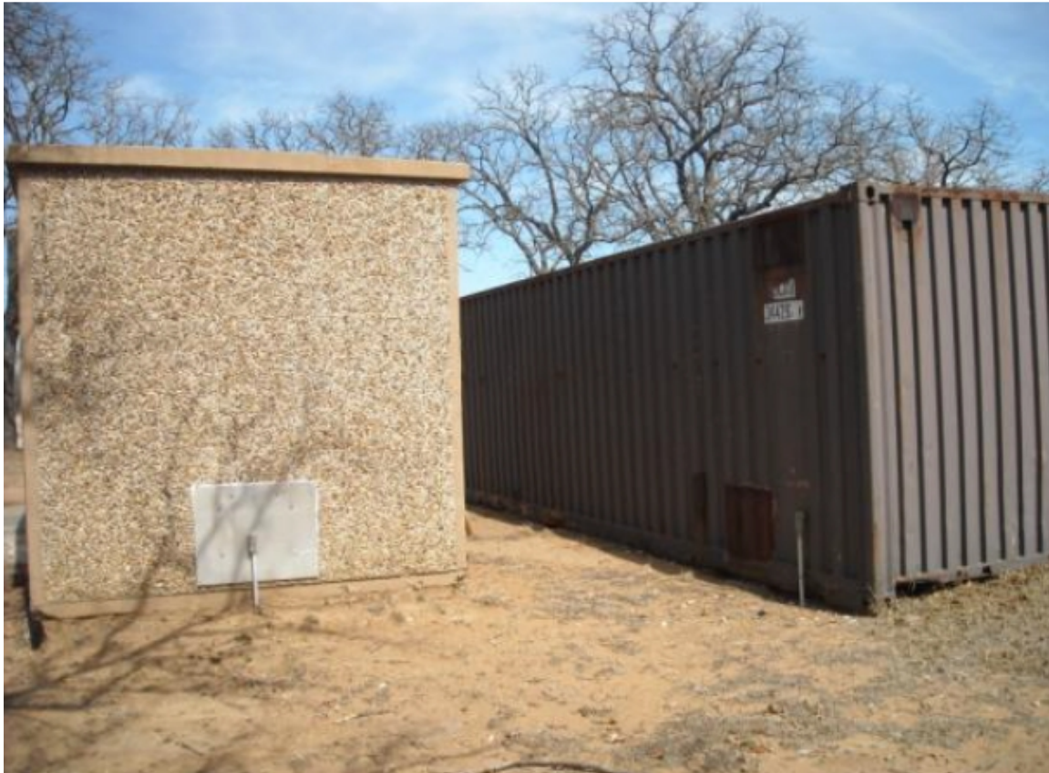
Figure 3-6 Proposed Site of Facilities: Building Labeled with Hazardous Materials Sign
