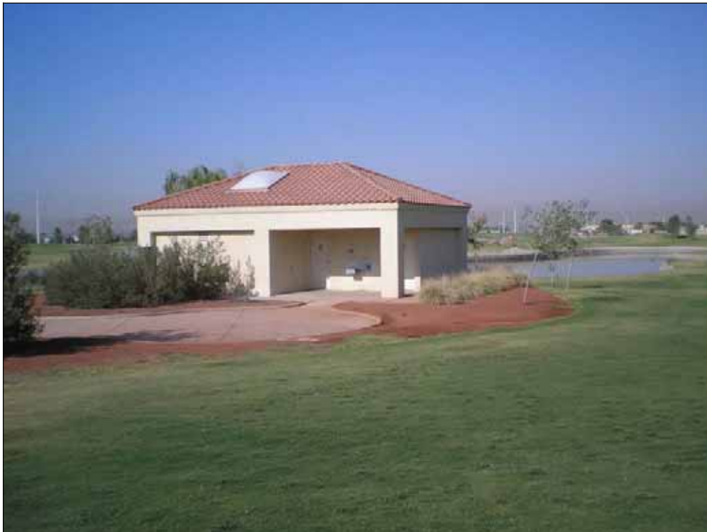
Photograph 16. Restroom facility on subject property
