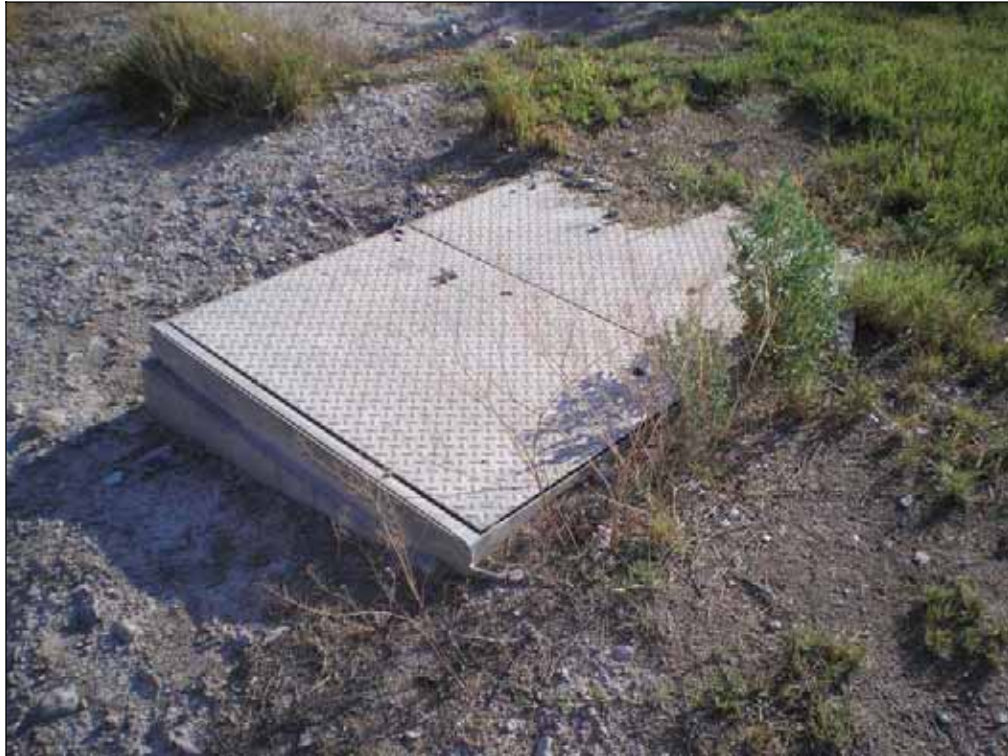
Photograph 9. Underground access at northeast subject property corner
