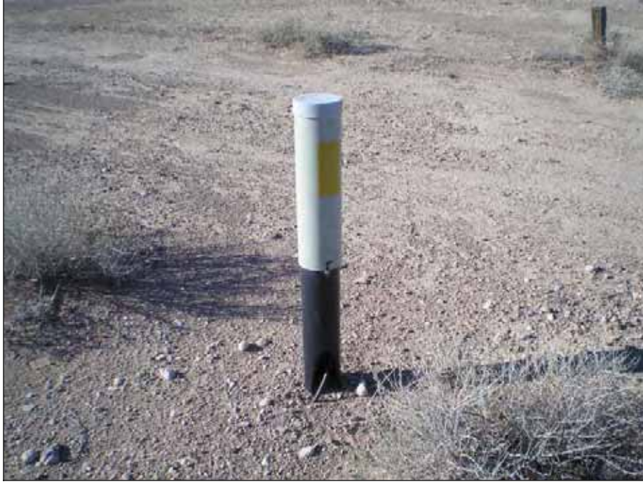
Photo 21. Telephone junction box on subject property
