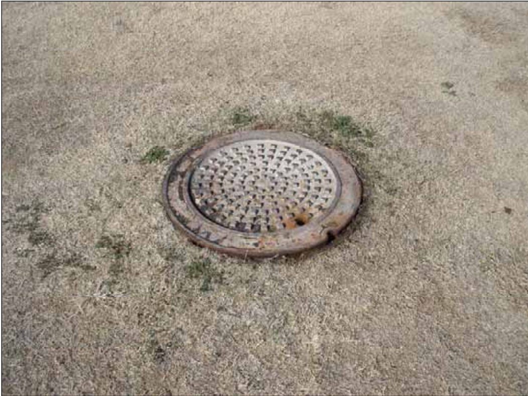
Photograph 11. Sewer access cover on golf course east of subject property
