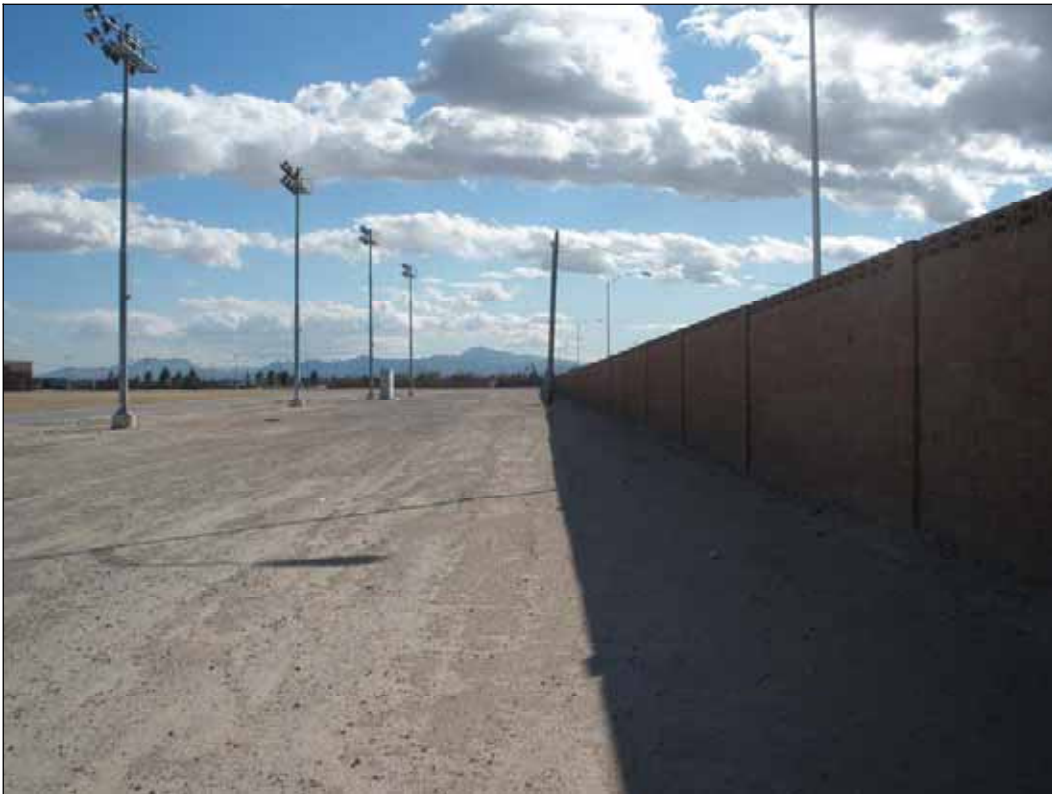
Photograph 14. South view of subject property from near the water tank
