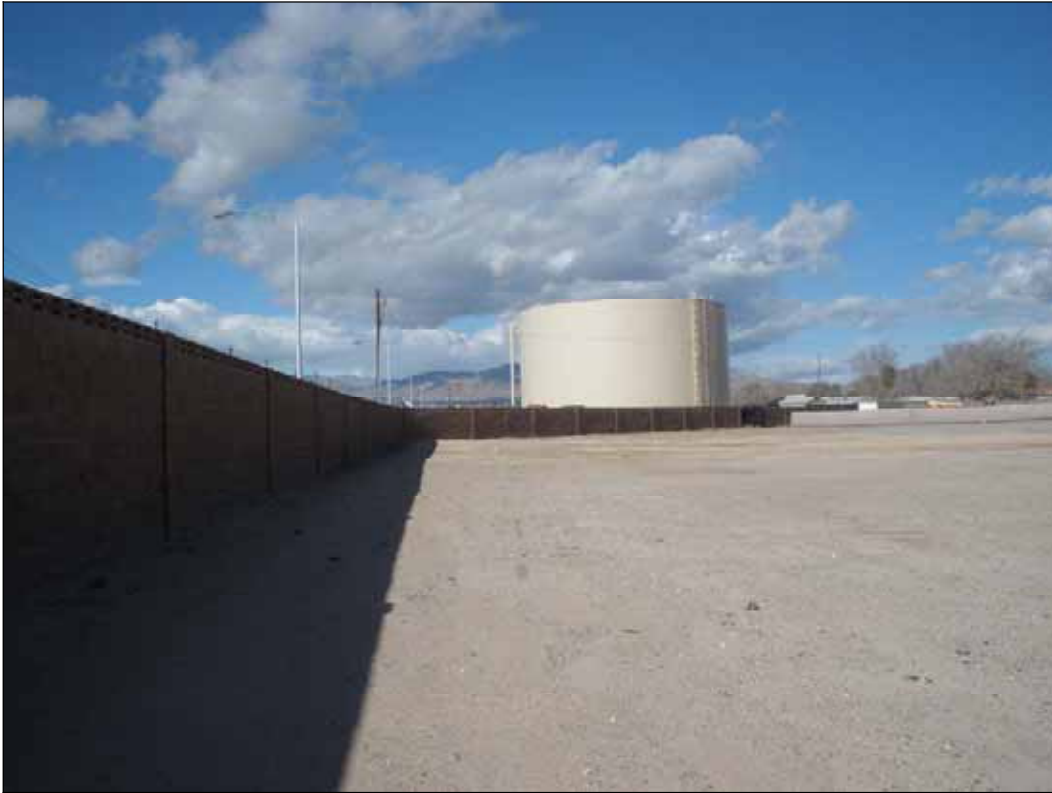
Photograph 13. North view of water storage tank adjacent to subject property
