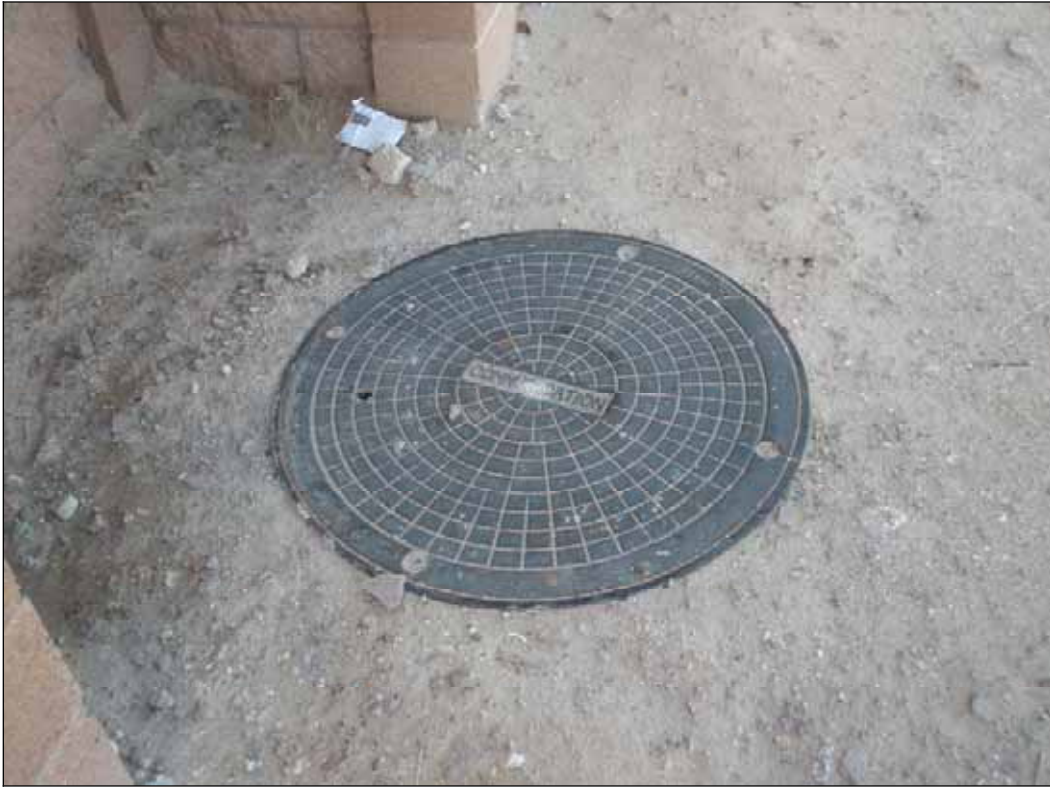
Photograph 17. Communications access cover on subject property
