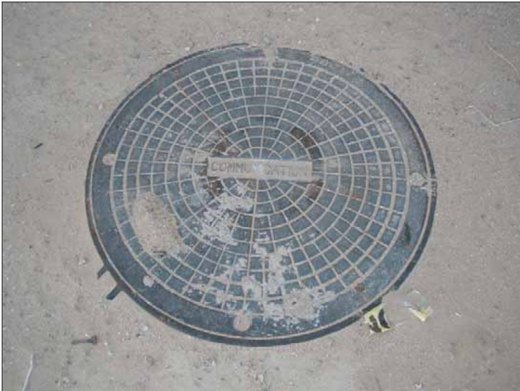
Photograph 15. Communications access cover on subject property
