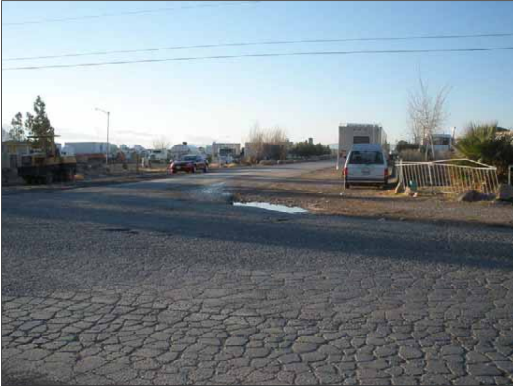
Photograph 1. South view along Betty Lane from subject property
