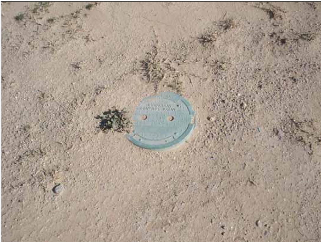
Photograph 10. Irrigation system valve on subject property
