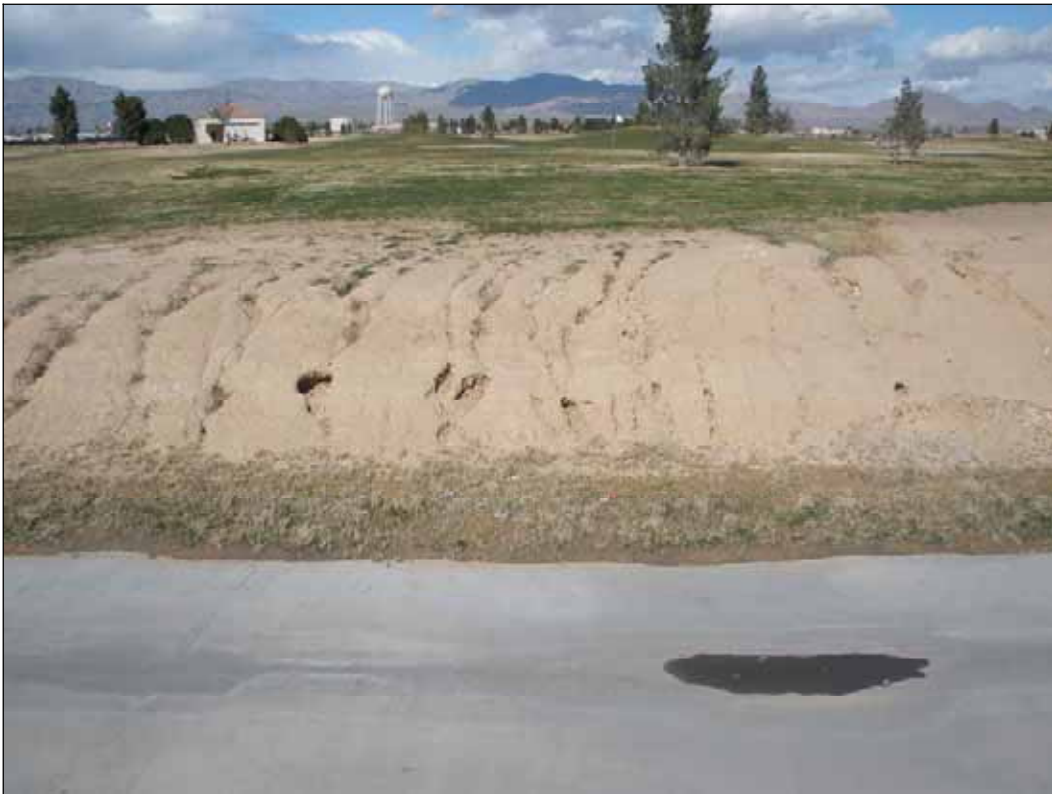
Photograph 4. North view of subject property at Sloan Channel crossing
