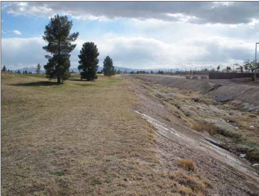
Photograph 12. South view of subject property from the Tyndall Avenue bridge
