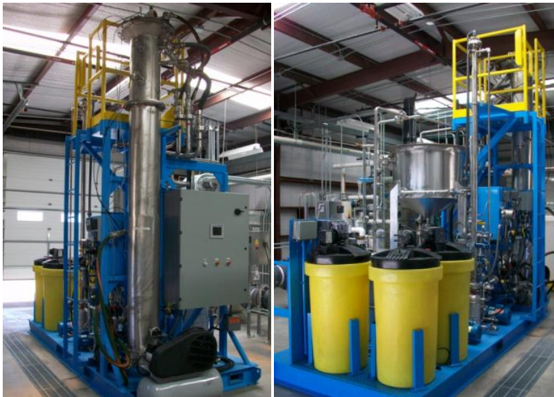
Figure 9. Photographs of the installed FBR system.
