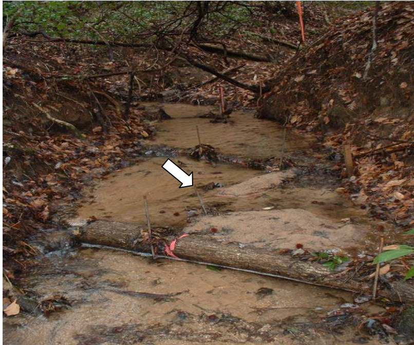
Figure 87. Photograph showing burial of instream debris dams by sediment, approximately 6 months after placement (K20, February 2004). Note almost complete burial of central log in the dam (shown by arrow) and generally low accumulation of organic matter (leaves, twigs) across the debris dam.
