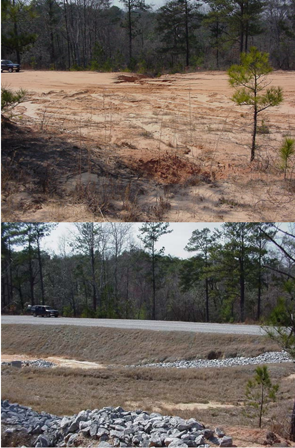
F3. Road was stabilized and banked. A sediment catchment basin was created and hillslopes were stabilized with vegetation and rip-rock. Project was completed in June 2005.
