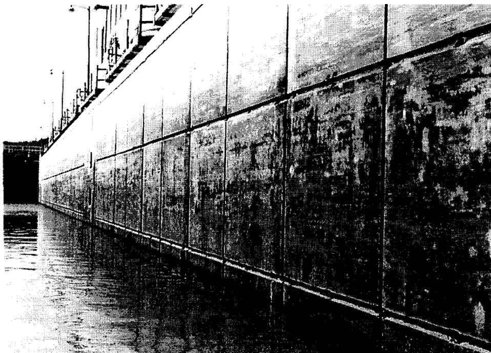
Figure 2. Precast lock wall panels
