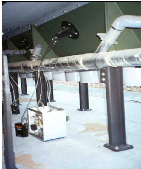
Figure 2. Twentynine Palms Test Setup.
