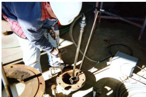
Figure 6. Top of the LRDP Being Installed in an 8-in Opening in a 50,000-gal UST at the Hunter Army Airfield.
