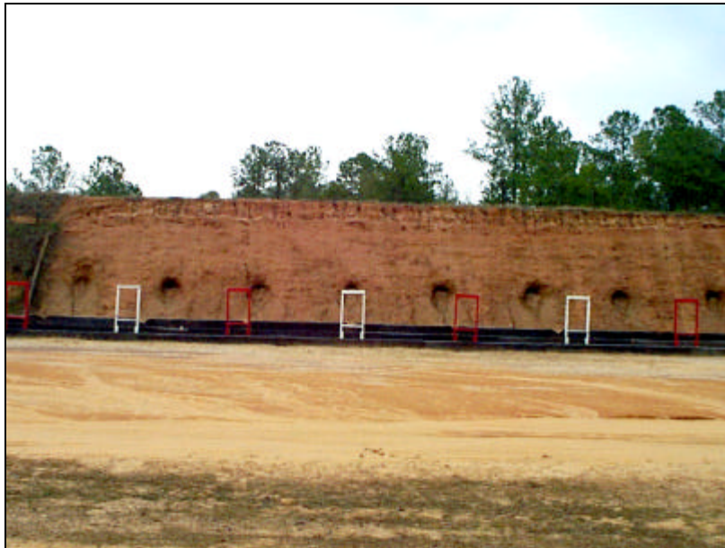
Figure 3. Small-Arms Range Berm
