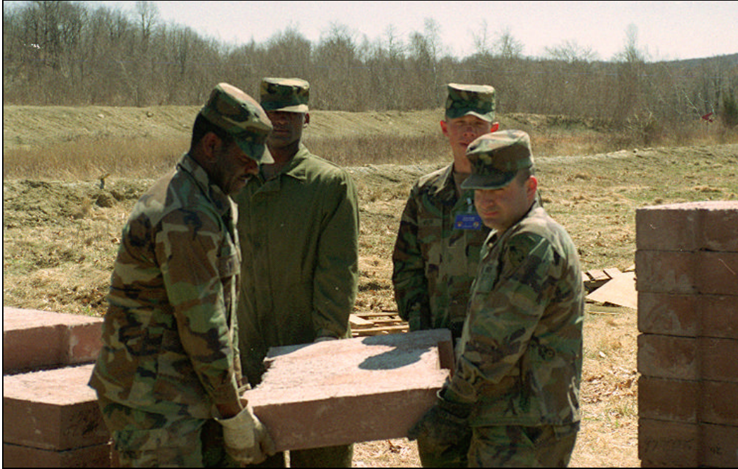
Figure 13. Four-Man Lift of 200-Pound SACON Block
