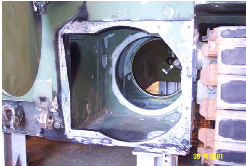
Figure 5.10: Seal Plate Mating Surface after Corrosion Removal
