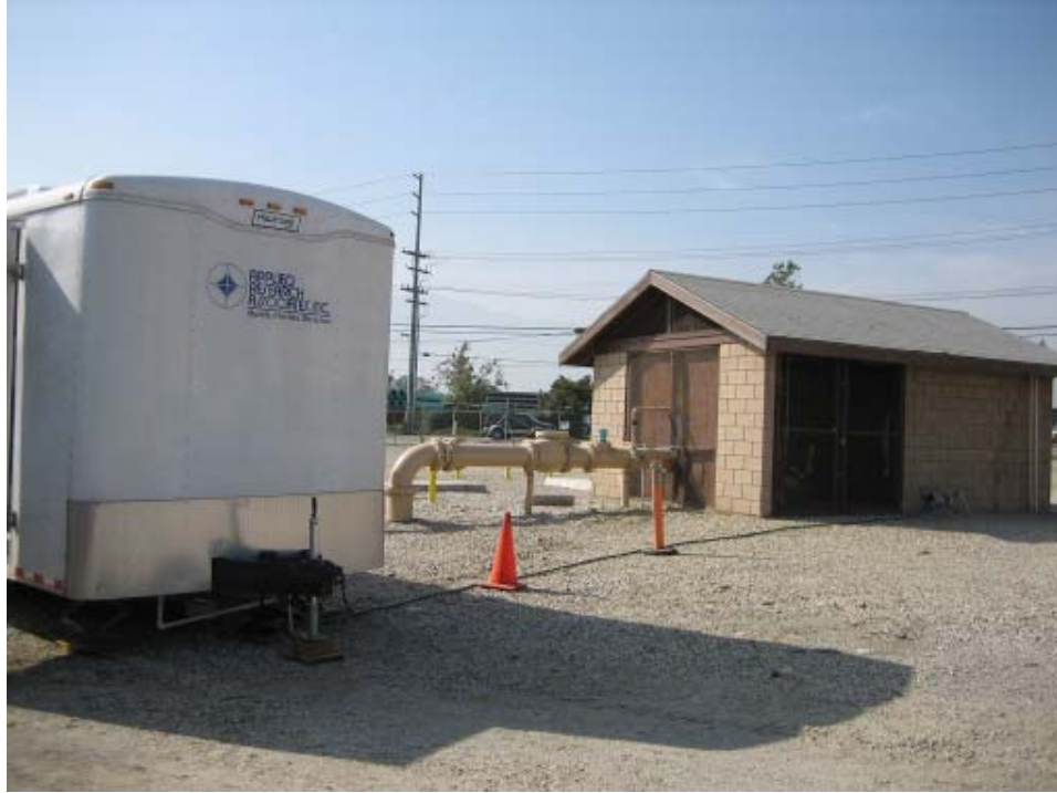
ARA Demonstration Trailer Beside Enclosure for Well F-17C in Fontana, California.
