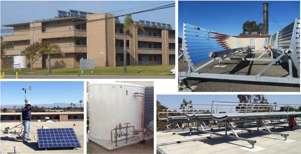
Figure 7: Photos from the installations at Port Hueneme and PRFTA. In addition to the SunDeck systems, a hot water tank, weather monitoring station and traditional PV reference panel are also shown.
