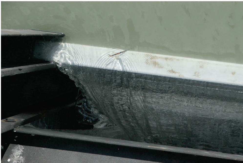
Figure 12. Plan view of composite weir boards DMMA M-5, Stuart, Florida.
