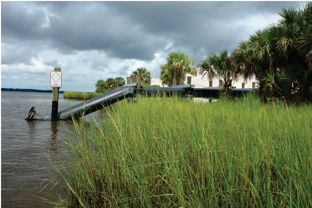
Figure 11. Elevated 30-in. outfall pipes minimize wetland impacts at Bartram Island Cell B2.
