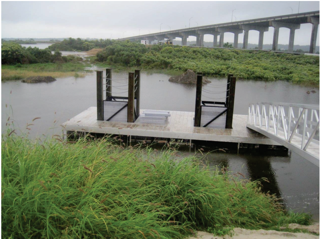
Figure 3. Bartram Island Cell F floating dock in use with composite weir boards removed and stacked on the dock's deck from two sides of each box riser.
