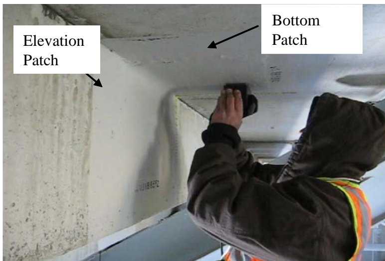
Figure 7. Inspection in progress.
