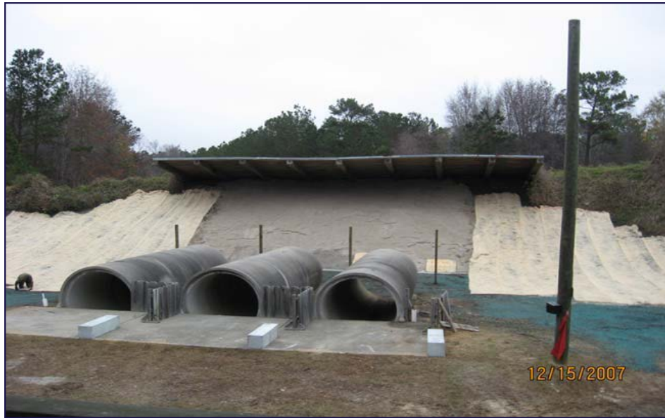
Figure 20. The completed impact berm enclosing the three experimental treatment lysimeters on the M60 range, CAFB.
