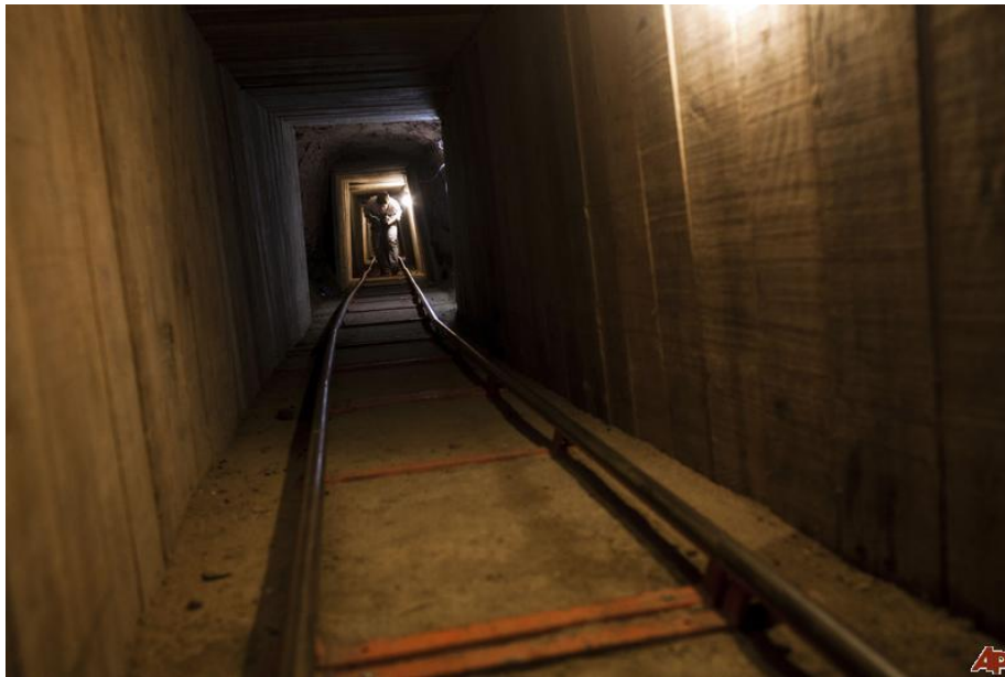
Figure 15. Tunnel between Tijuana and San Diego. 247
