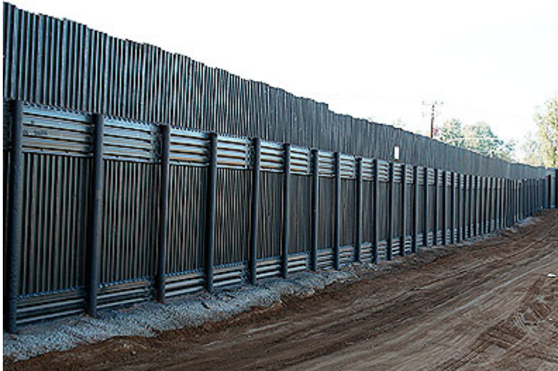
Figure 12. Landing mat fence in El Centro 244
