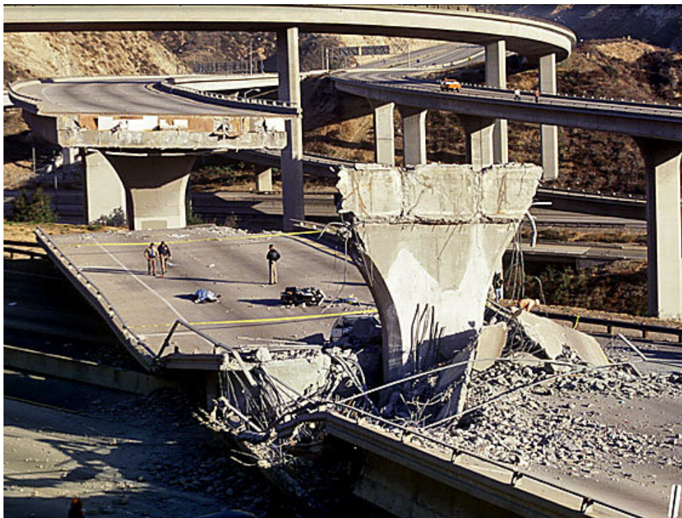
Figure 4. Northridge earthquake freeway damage (from Mehmet and Brown 98)
