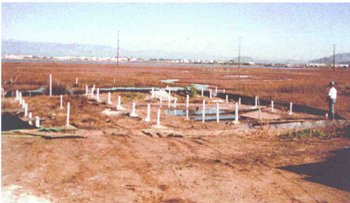
Figure 15: Test Cell #1 Electrode Wells Installed
