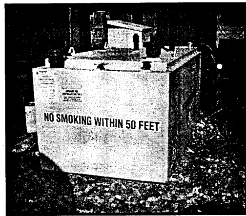
Figure 4.2-3 - A 30-Kilowatt Diesel Powered Generator and 500 Gallon Auxiliary Tank.
