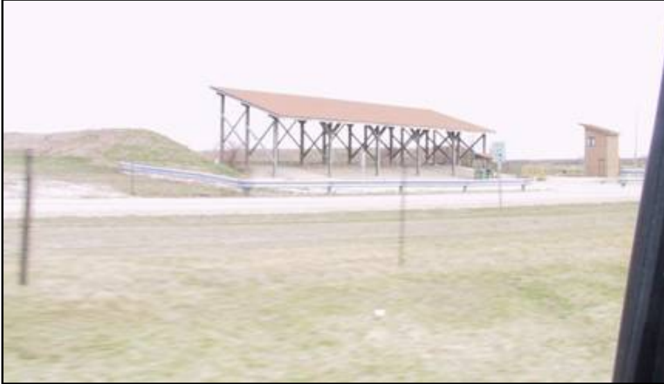
Figure 10. Photo of a small arms range at Marseilles Training Area featuring a covered firing line and safety berms at the sides of the range and behind the targets.
