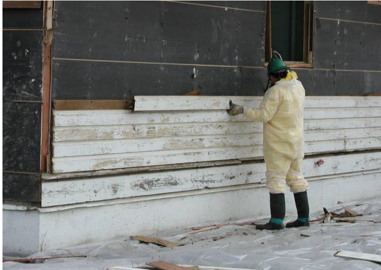
Figure 4.1. Piece-by-piece siding removal.
