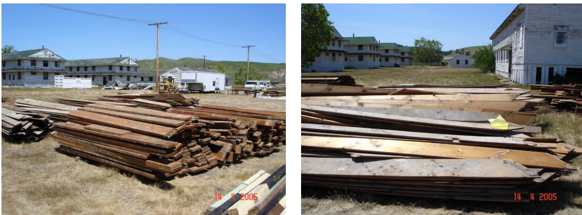
Figure 4.5. Salvaged framing (left) and subfloor lumber.
