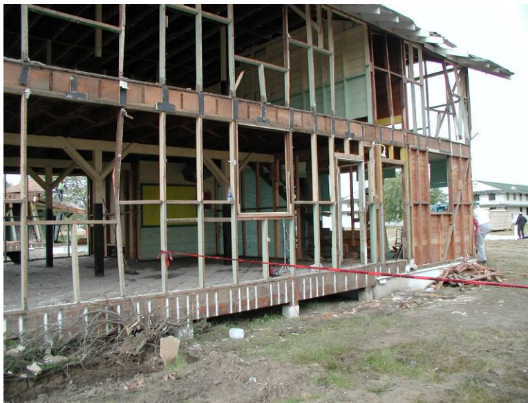
Figure 4.2. Siding removed; ready for deconstruction.
