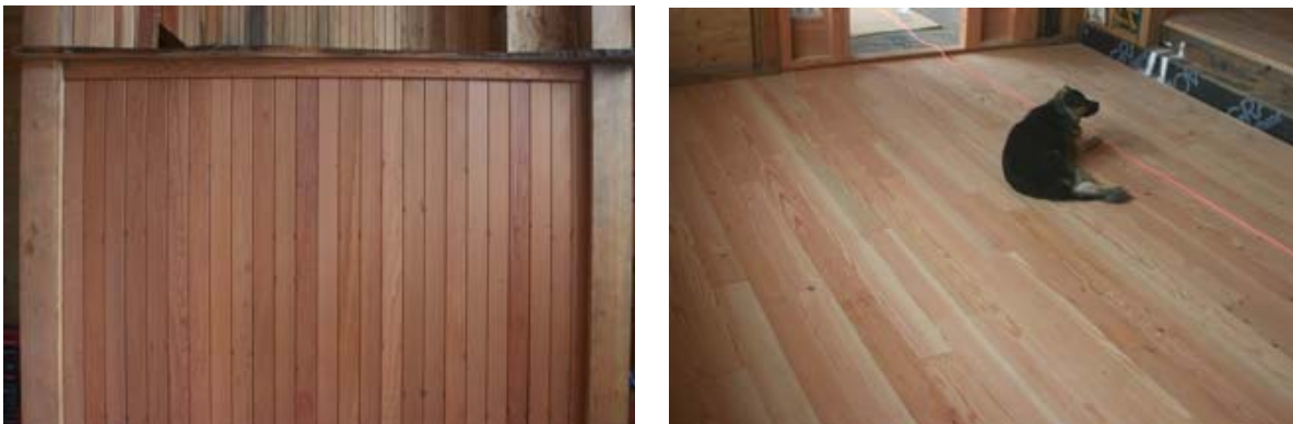
Figure 4.6. Redwood paneling (left) and Douglas fir T&G flooring (right) milled from a portion of salvaged siding from the Camp Roberts
