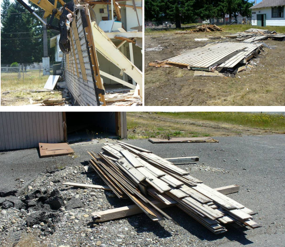
Figure 4.16. Highly efficient panelized deconstruction, disassembly, and siding removal at Fort Lewis.
