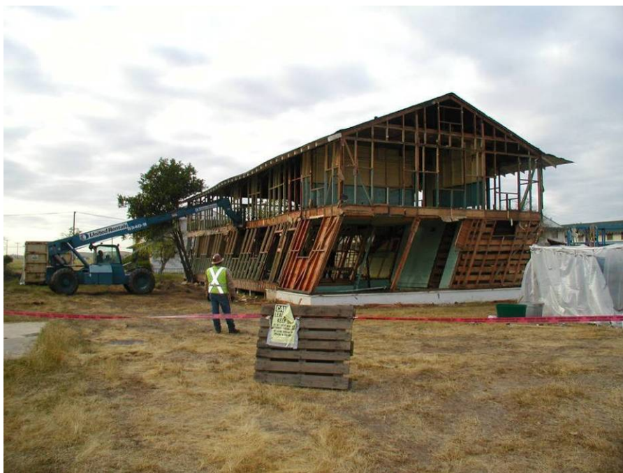
Figure 4.4. Building being pushed over for further deconstruction.
