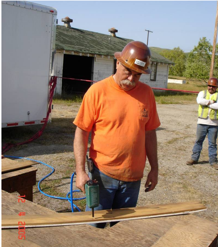
Figure 4.3. Denailing reclaimed siding using pneumatic tool.
