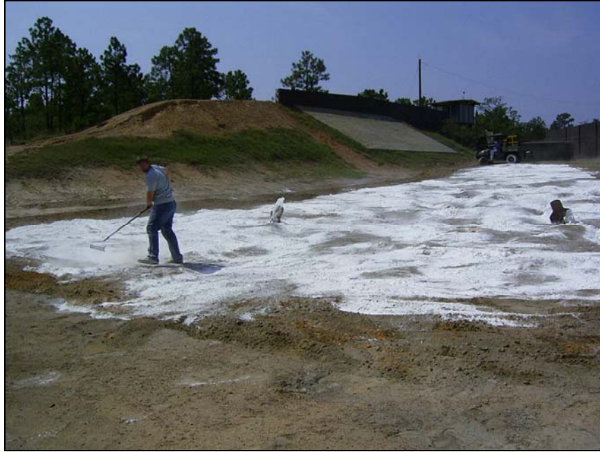
Figure 6. Applying \text{Ca}(\text{OH})_2 by hand
