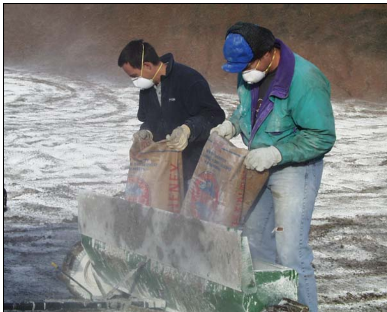
Figure 14. Staging bags of lime to apply to the treated HGR bay
