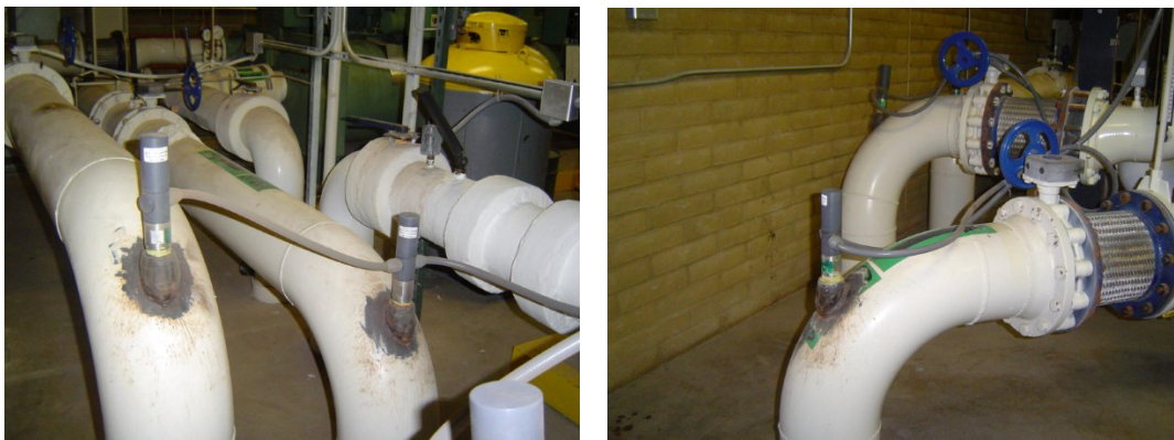
Figure 5. Capacitor rods inserted into 1.5 in. thread-o-let fittings in CWS & CWR lines at Fort Huachuca SCP.
