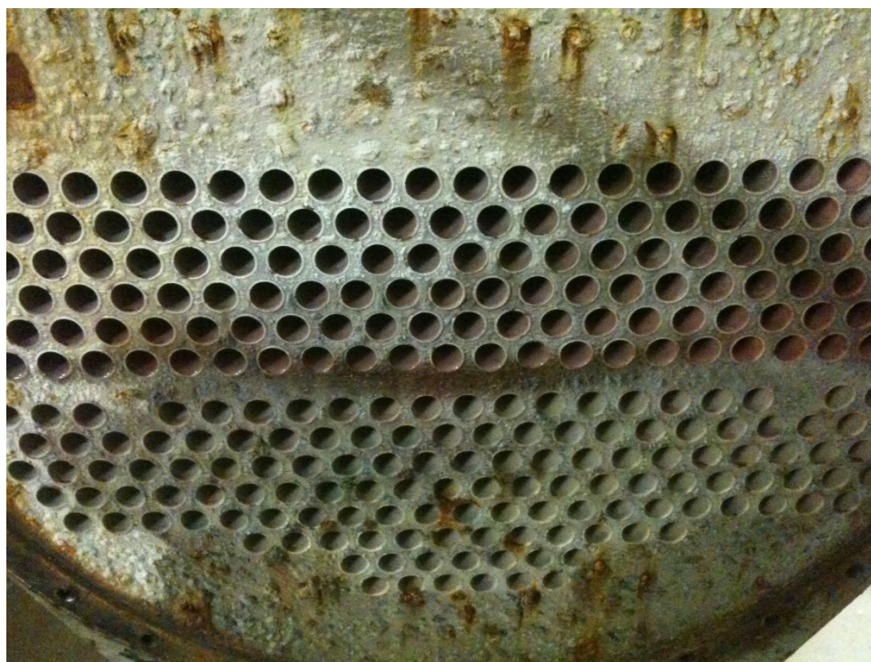
February 2, 2010: Fort Irwin Bldg 273 (Control) – scale visible on tube surfaces. Thicker layer on bottom tubes (second pass) than on the top half tubes (first pass).
