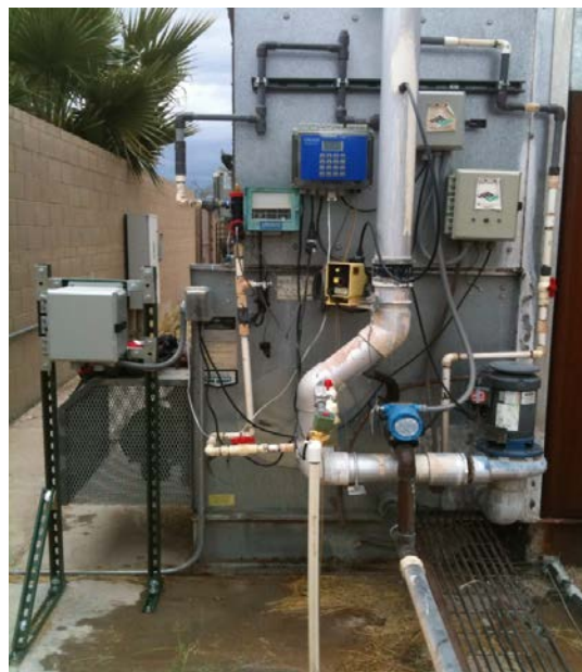
Figure 11. Zeta equipment mounted on evaporative condenser at Davis-Monthan Building 2301, Fitness Center.
