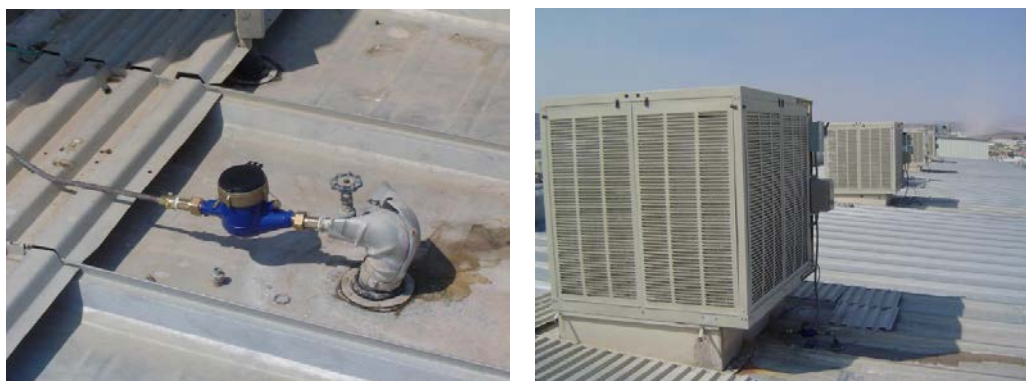
Figure 18. Fort Irwin Building 873 (Zeta Rod test site): water meter installed on swamp cooler (left); swamp coolers on the roof (right).
