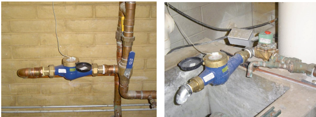
Figure 6. Two-inch water meters in makeup water line (left) and blowdown water line (right) at Fort Huachuca SCP.
