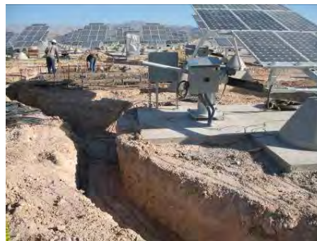
Trenches for underground conduits
