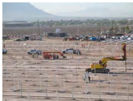
Clearing land and drilling footings
