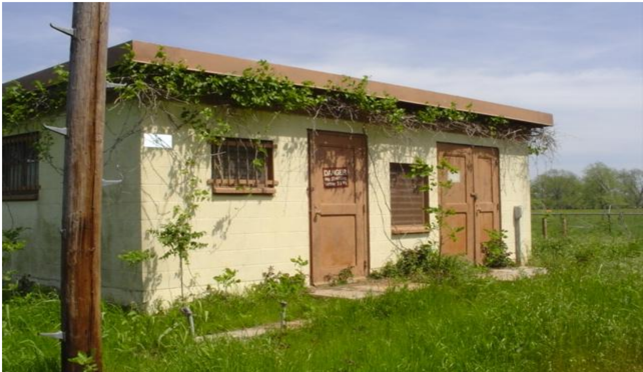
Figure 1 ILS Middle Marker Building
