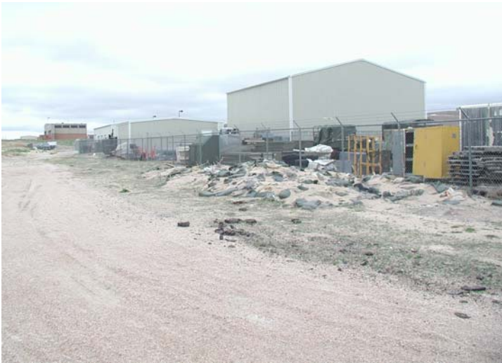
Photograph 9: Building 1002 Looking southeast at AASF
