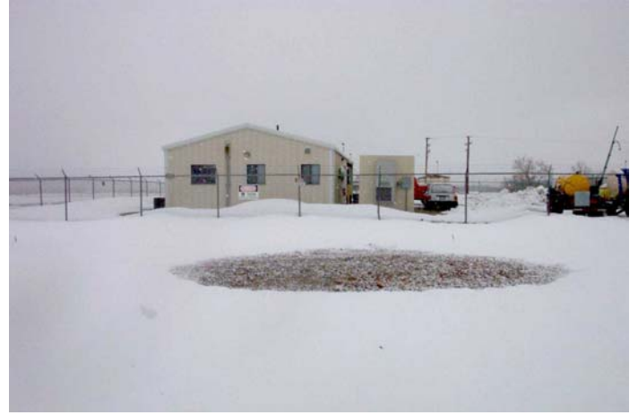
Photograph 2: Building 306 looking east
