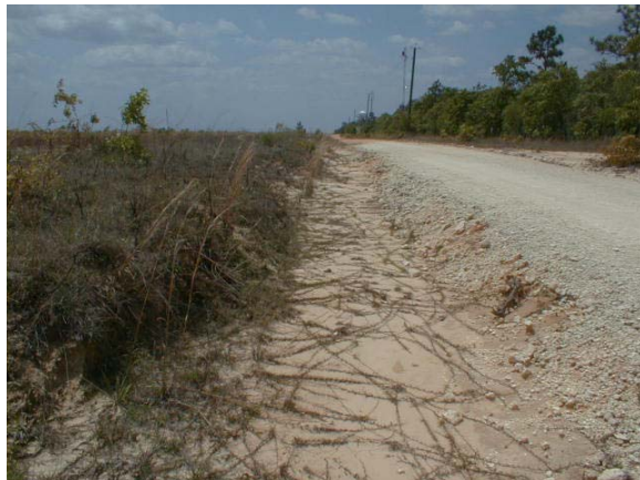
3-42a. Upslope view of the roadside ditch
