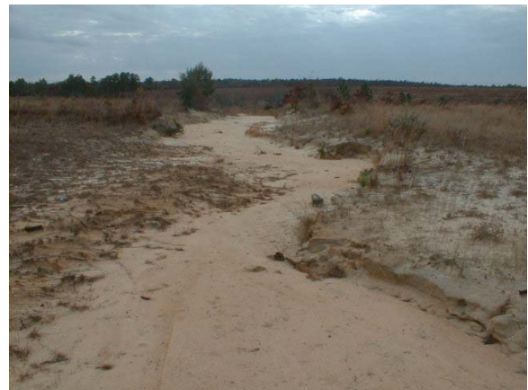
3-37f. EIA-1 access road that functions as a gully conveying runoff and sediment to the stream slope
