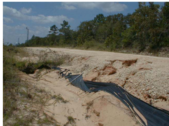
3-42d. Roadside ditch outfall August 2001
