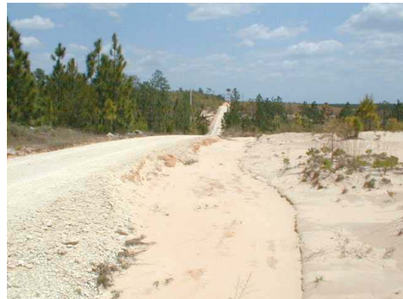
3-42b. Downslope view of the roadside ditch
