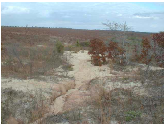
3-40c. Road/stream slope sediments are delivered directly into the Oakie Creek stream channel
