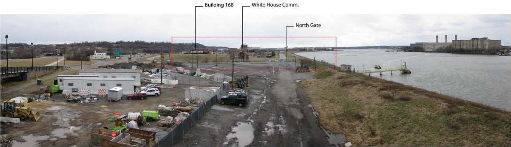
Panoramic View from South Capitol Street Bridge
