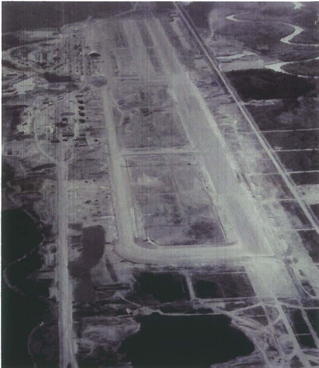
Figure 3-1 – Eielson Under Construction, circa 1951.
