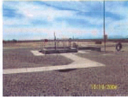
Photograph 2: View of the septage disposal basin at the wastewater treatment plant.
