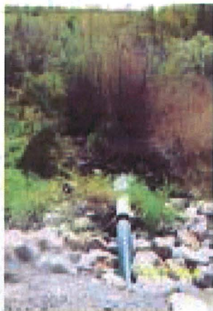
Photograph 11: View of the 6-inch forcemain outfall at Lagoon C.
