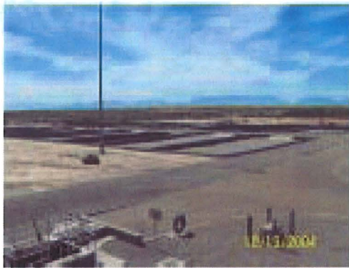
Photograph 7: View of the sludge drying beds at the wastewater treatment plant.
