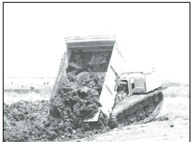
Placement of dredged material for habitat restoration (Photo by USACE).
