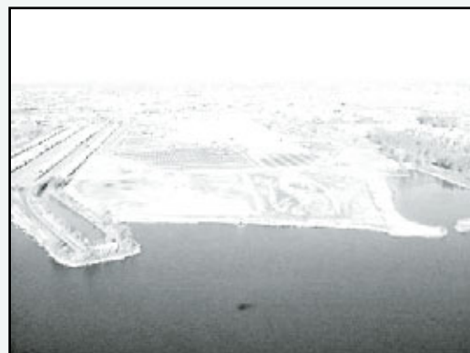
(Photo by USACE)
