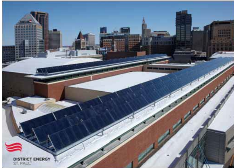
Figure 4. Solar water heaters installed on a roof (WBDG 2011).
