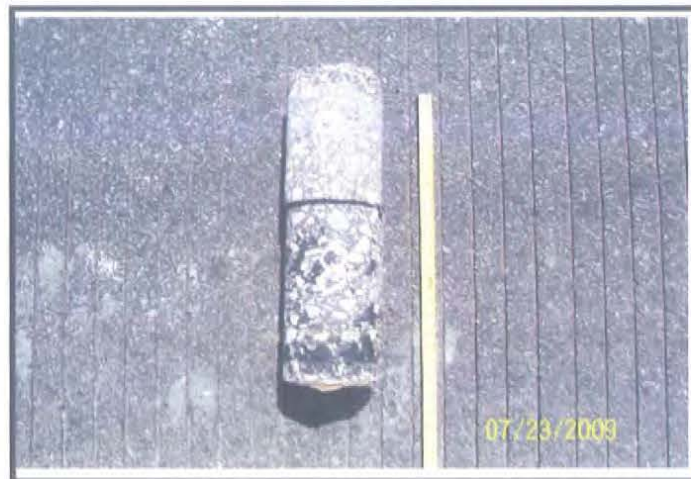
Taxiway C Core No. 8
