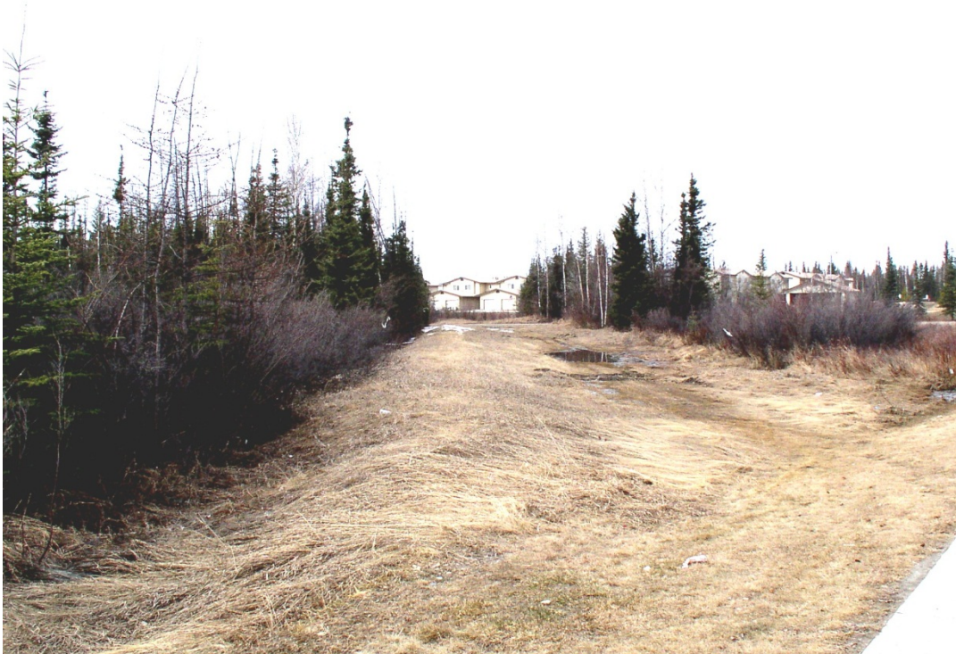
Figure 3-3 – Right of Way of Existing Direct Buried Utility Lines
