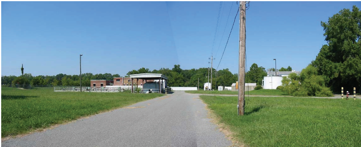
The Big Bethel Reservoir Water Treatment Plant Site
