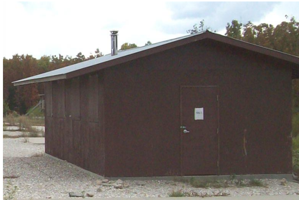
Figure 33. Structure with windows to allow natural ventilation.
