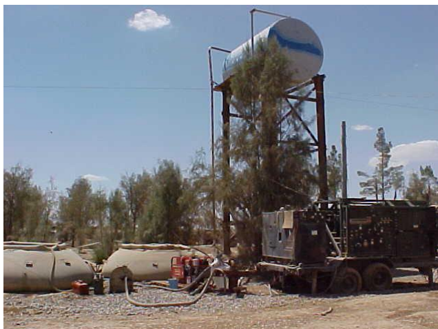
Figure 10. Elevated tank at water supply point.
