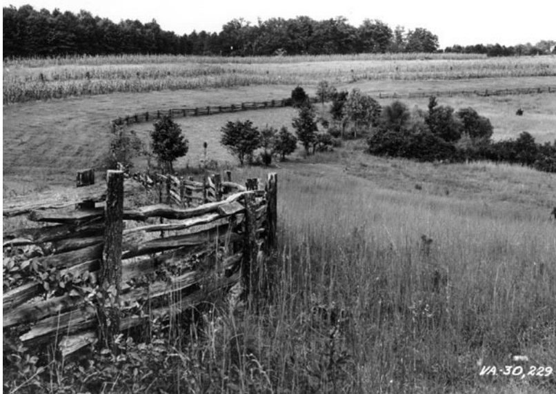
Figure 19. Split-rail fence, 1938 (National Agricultural Laboratory).
