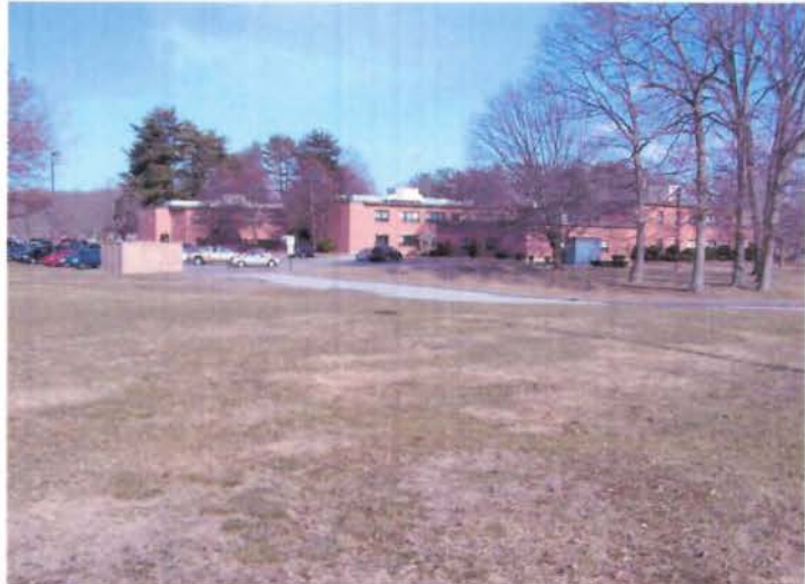
Existing Bldg 1600 to be demolished and replacement Acquisition Management Facility to be constructed within same parcel
